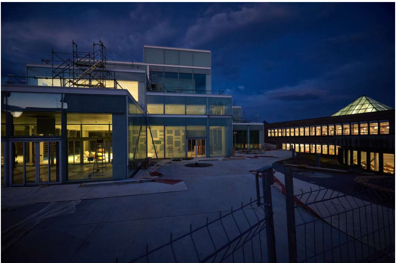
Current state of the building site. (zVg)
